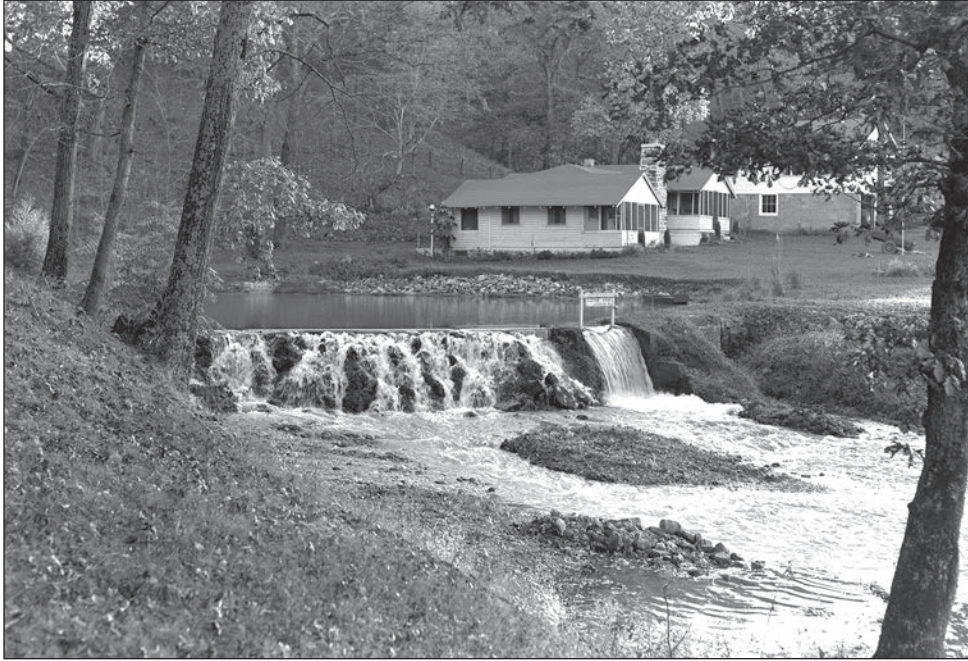
Water gushes over a dam and spillway at Slabtown Spring, discharging 10,000,000 gallons per day from the base of a ridge. Photograph by Gerald Massie, circa 1950. Courtesy of the Missouri State Archives.
